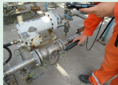
VOC漏えい測定(Leak Detection)
